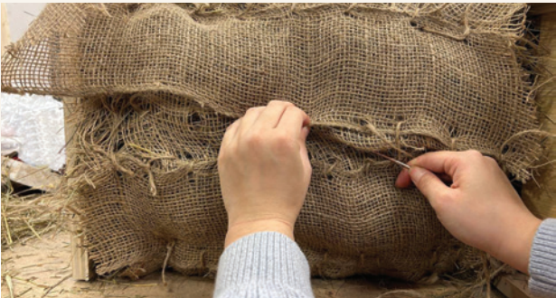
Wall Assembly R-29.04 lime plaster finish (stabilized) burlap 4" straw insulation burlap 10mm grass batt insulation burlap 2"x4" studs at 2' O.C. 4" straw insulation burlap
